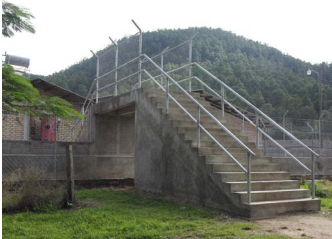
Overcrossing leading to the newly built workshops
