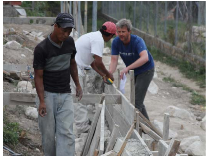
Construction of a fence on the vocational site
